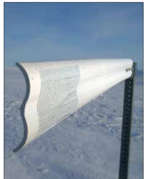
When installed, the delineator post or "arm," projects horizontally from the shoulder, above the roadway, and is capable of rebounding when struck. The delineator also provides excellent reflectivity at night.
