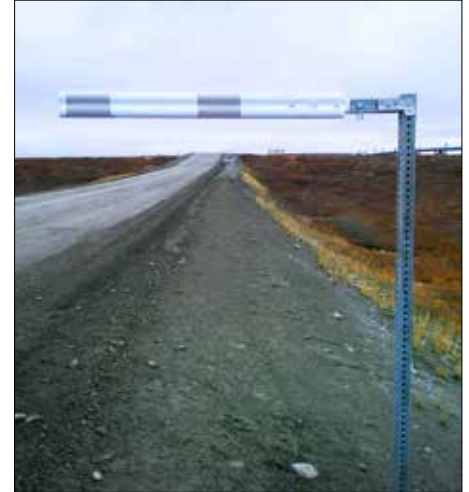
The "Dalton Delineator" consists of an extruded roadside delineator profile mounted to a second extrusion – a special, flexible coupler.
