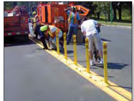
Installing Interstate Grade Curb
