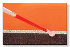
The bottom panel is 1.5" from the ground and acts as a detectable edge for pedestrians using canes.
