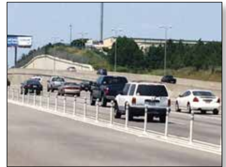
City Post SM Surface Mount I-85 Express Lanes – Atlanta, GA ADT: 260,000 – Speed: 70 MPH
