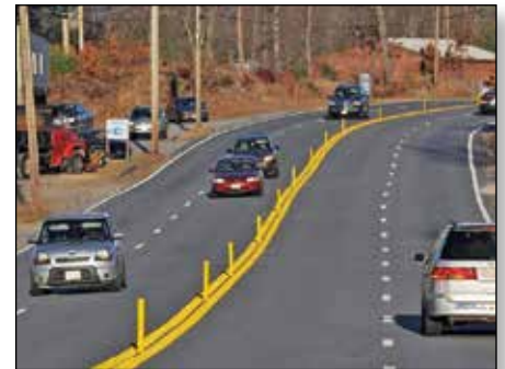
Separation of opposing traffic on dangerous curves
