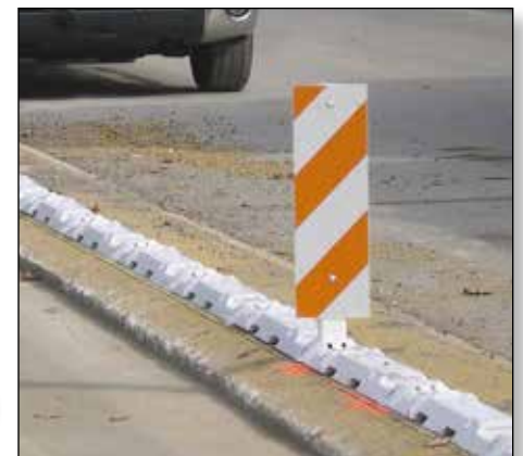
Work zone panels can also be used with temporary or permanent curb installations
