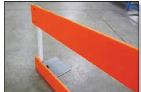
The top and bottom barricade panel share a common vertical face and nothing protrudes into the walkway.
