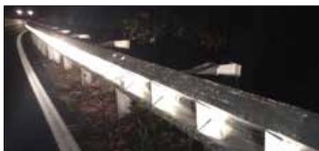
Reflective guardrail markers create bright delineation, creating safer roads and safer driving conditions.
