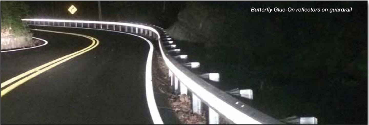
Butterfly Glue-On reflectors on guardrail
