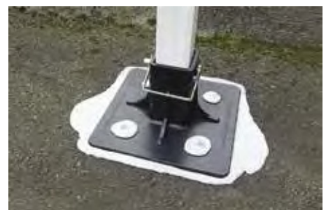
Quick Release Pin base installed with epoxy
