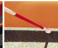
The bottom panel acts as a detectable edge for pedestrians using canes
