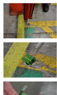
**Backfill the flights of the 4" cup with adhesive prior to installation.**
