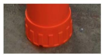
Once the adhesive is fully cured you can remove the City Post from the anchor cup. If the steps are followed correctly and in sequence you should have an installation that looks very similar to this.
